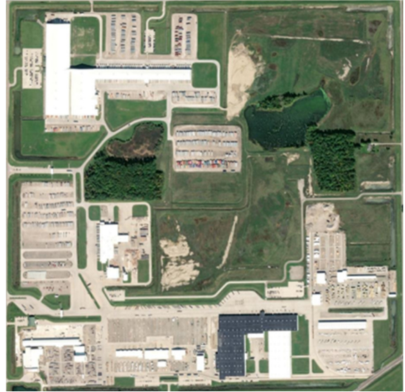
Menards Distribution Center
